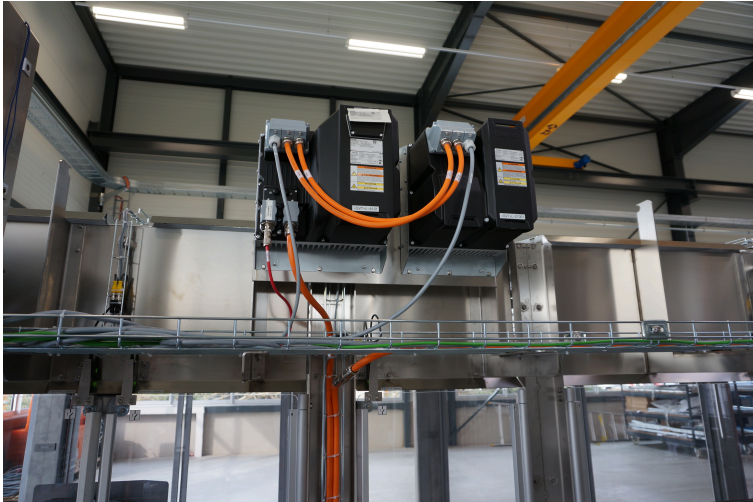
Control cabinet-free: The decentralized IndraDrive Mi drive solution allows a modular construction and reduces cabling thanks to serially laid hybrid cables. (Image source: WDS)
