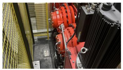
The two roller drives at Freudenberg Sealing Technologies each power 55 kW and use a Hägglunds CA100 hydraulic motor with a rated torque of 25,000 Nm and a nominal speed of up to 23 min-1. (Image source: Freudenberg Sealing Technologies)
