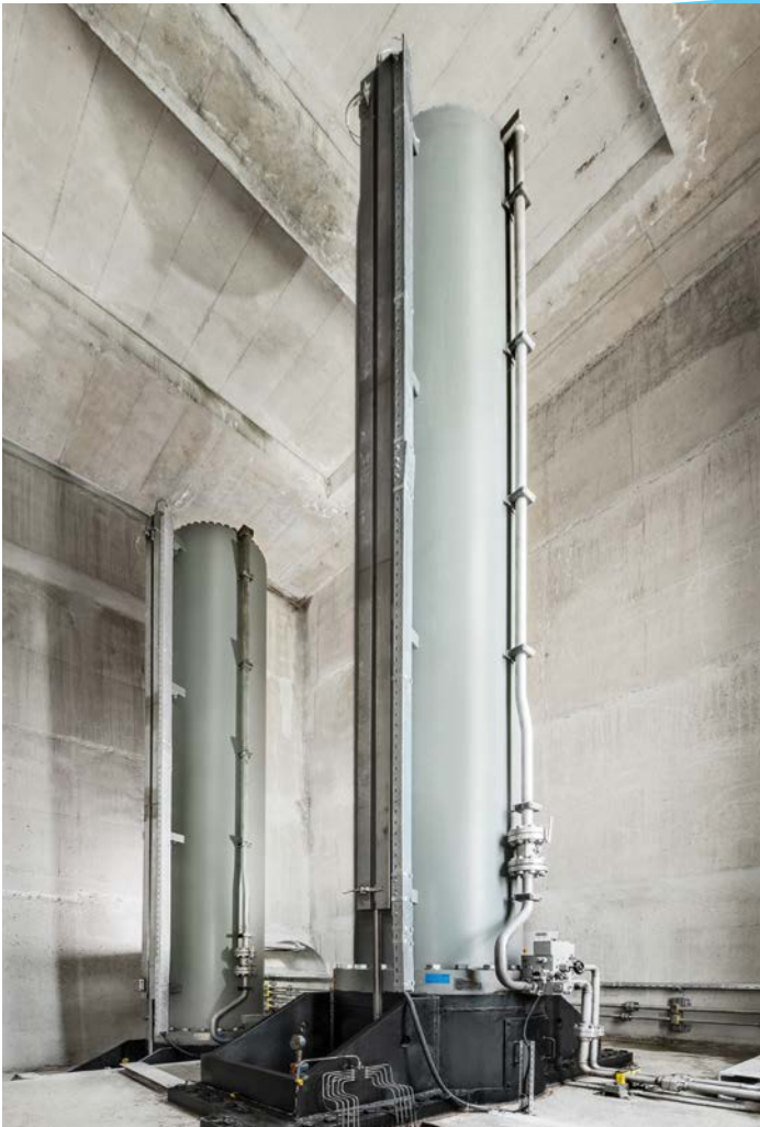
▲ Outlet gate (orifice) Cylinder piston Ø 900 mm Cylinder rod Ø 360 mm Stroke 6,000 mm Max. pulling and pushing force 12,000 kN
