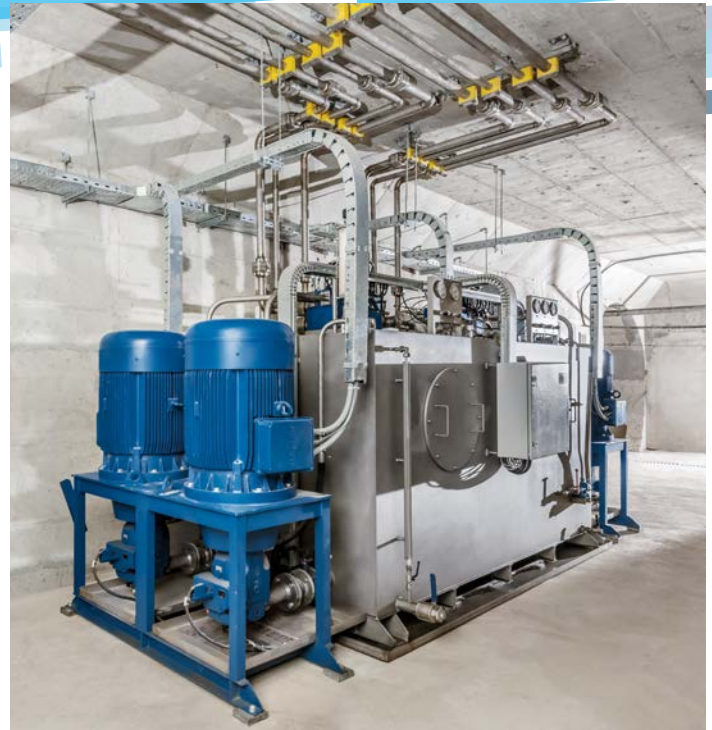
▲ Power unit for outlet gates
