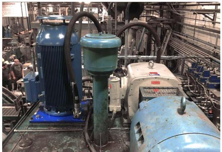
The image shows the space savings of the new pump configurations: the right side of the photo shows the legacy, horizontally installed pump and power unit, the left side shows the vertically installed new power unit; the pump itself is installed in the reservoir.
