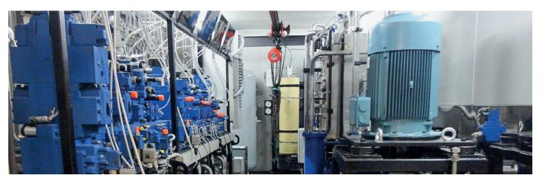
Tata Steel: Ready-to-connect hydraulics containers with the entire drive and control technology
